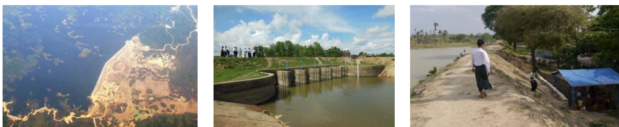
Figure 4-19 Catching rain in the wet monsoon and store for the dry season in numerous reservoirs throughout the dry zone (left), in irrigation canals in the Delta (middle) and in communal ponds with concentrated tap point at the low end of the dam (right).
