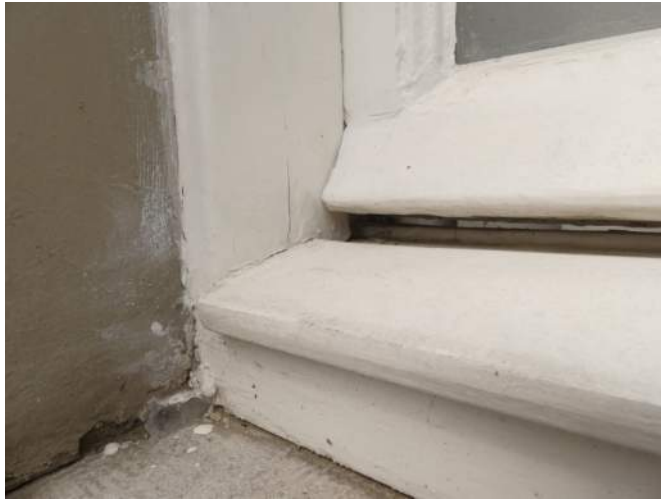
Afb. §46.21.13, barstjes in verf, beletage
