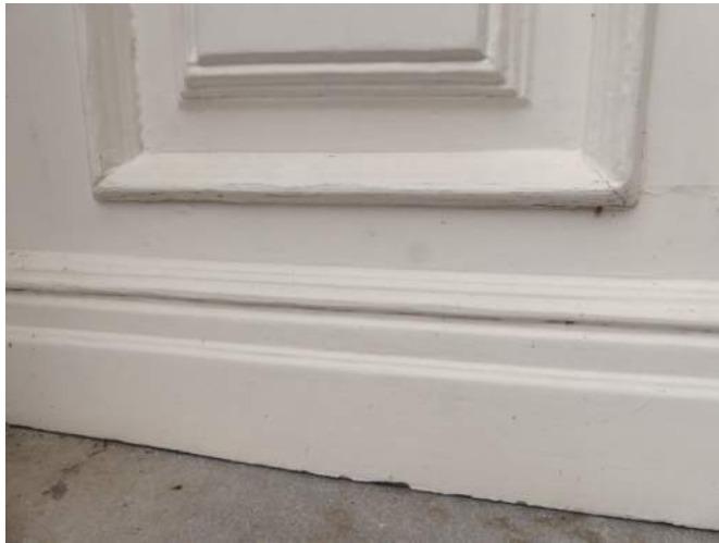
Afb. §46.21.15, barstjes in verf, beletage
