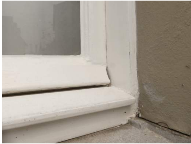
Afb. §46.21.14, barstjes in verf, beletage
