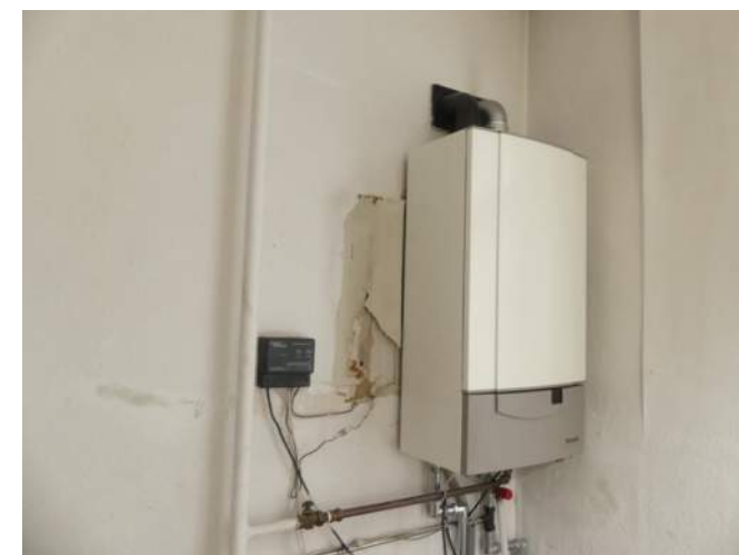
Afb. §60.01, cv-ketel in toren
