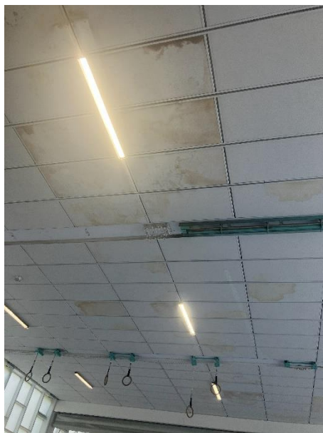
Picture 26: Plafond gymzaal
