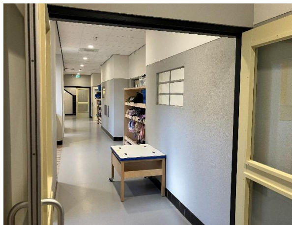
Picture 4: Brandwerende scheiding
