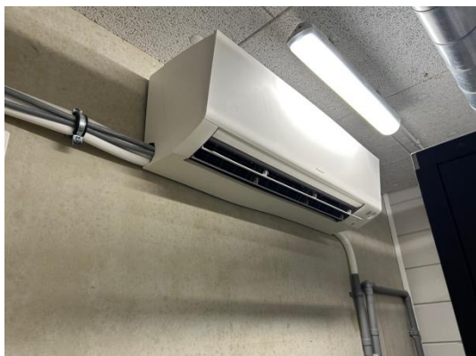
Airconditioning serverruimte
