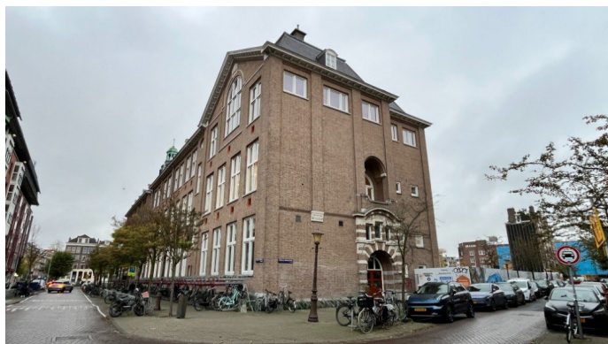
MLA, corner Nicolaas Maesstraat (I) and Pieter de Hoochstraat - new extension under construction on the right
