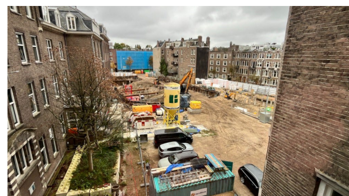
New extension (right) under construction
