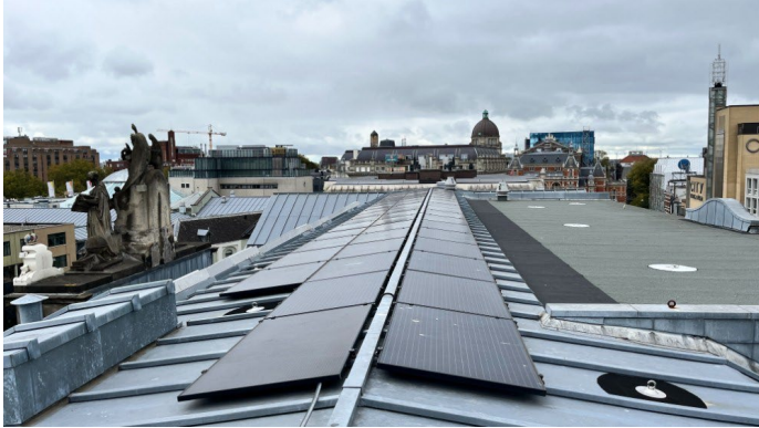
Building No 29, roof
