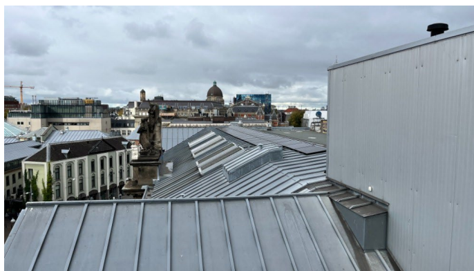
Building No 29, roof
