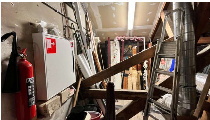
Attic, used for some storage. Note the fire extinguisher, hose reel and fire alarm button.
