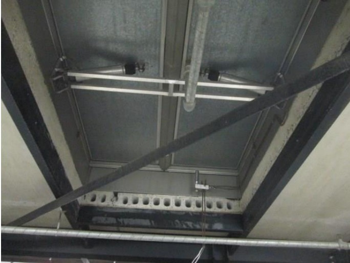
Smoke hatches above the stage
