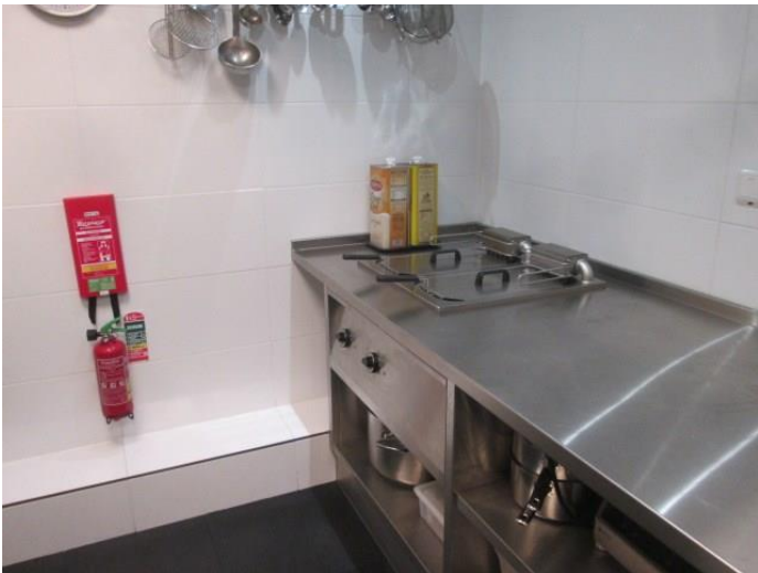
One of the three kitchens with deep fat fryers
