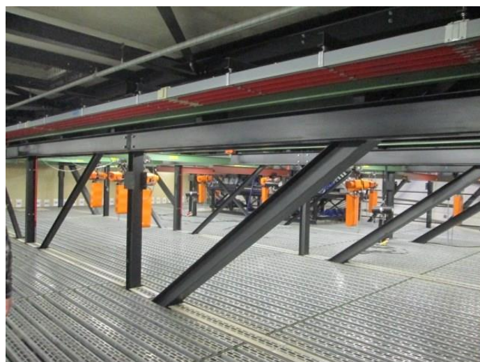
The top construction above the stage
