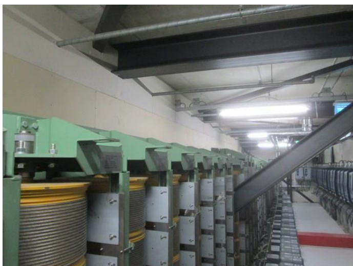
Hoists to lift curtains and decorations at the stage
