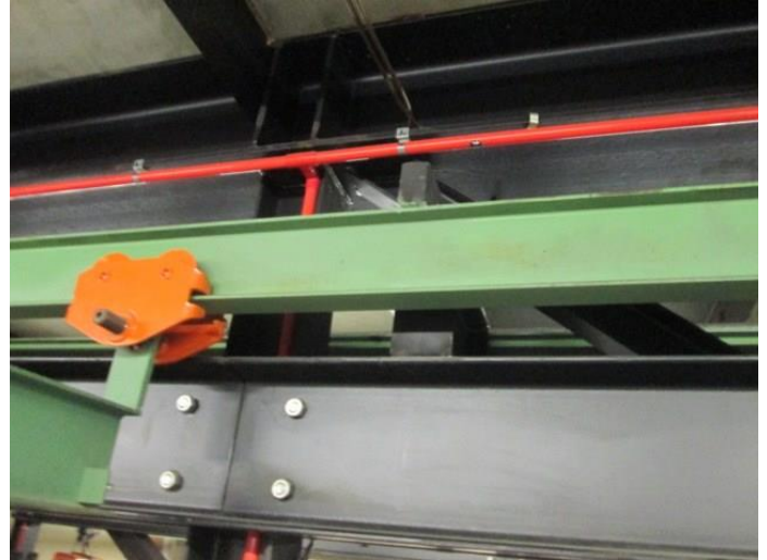
Aspiration detection above the stage
