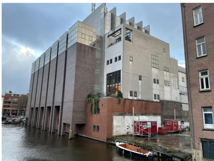
The rear of the building (new construction)
