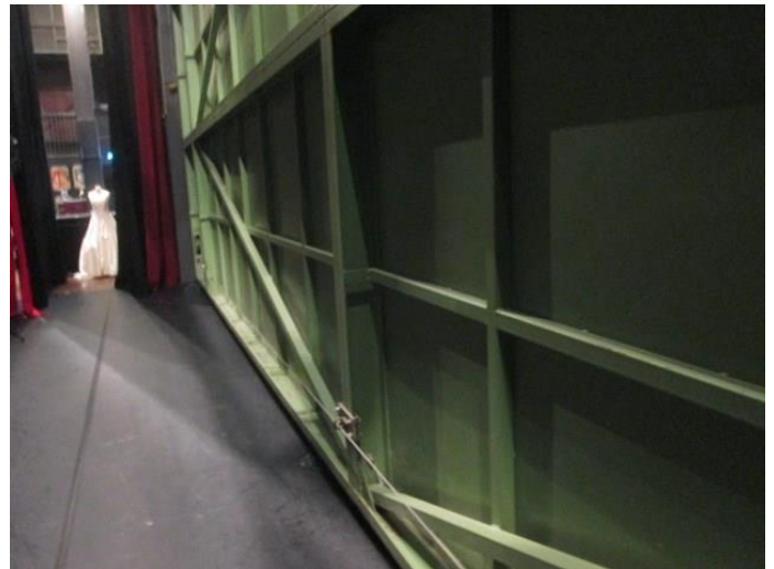
A steel shutter between the stage and the audience as fire retardant barrier.
