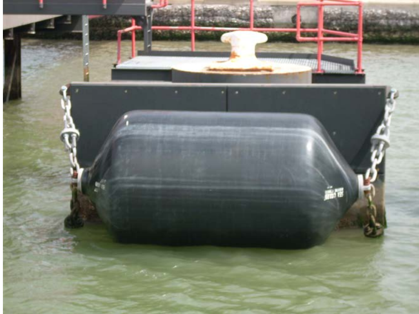
Alternate backing surface requiring larger fender end fittings
