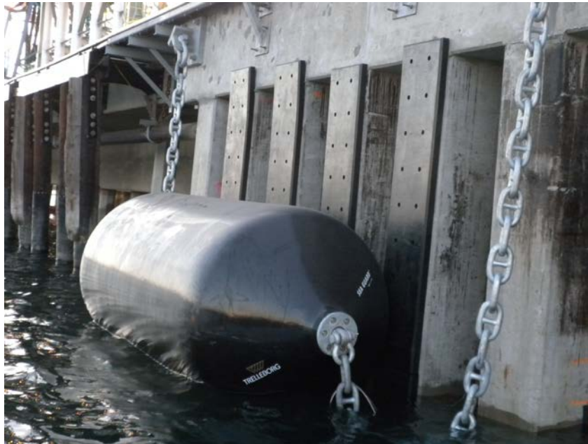
Typical two-point mounting configuration
