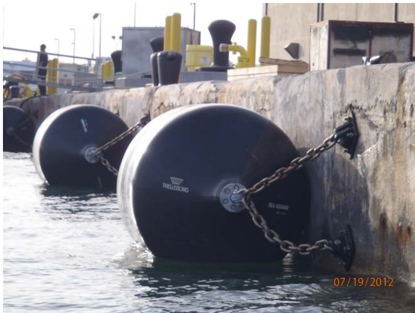
Typical four-point mounting configuration
