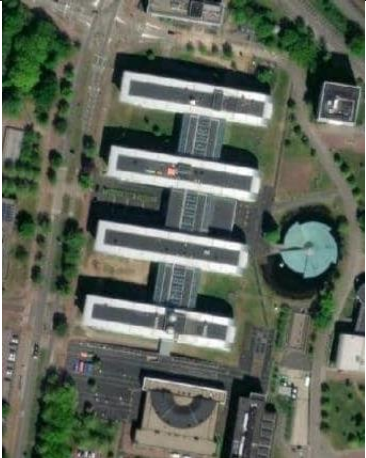
Overview of the Huygens building. At the right (green roof) is the MRI building. This is at basement level and just a minor part is above the pond/grade level) Therefore this exterior exposure is classified as separate fire area.
