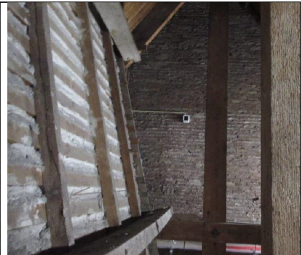
The attic above the previous chapel with beam detection
