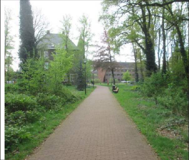
The rear of the building
