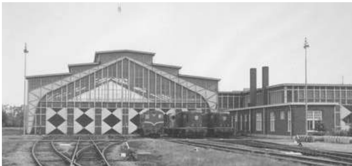
Locomotiefloods Roosendaal &lt;HUA&gt;
