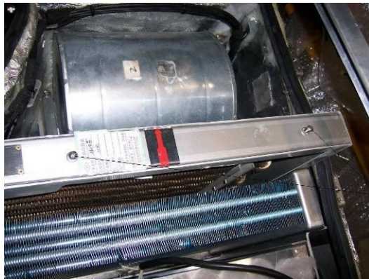
Figure 5.77 Loosen the bolts of heater cover
