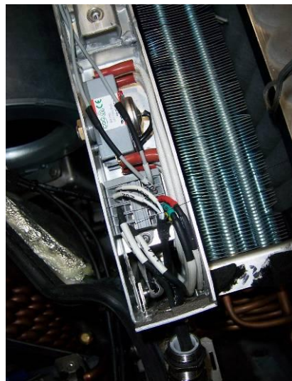
Figure 5.78 draw out the cables from the terminal block
