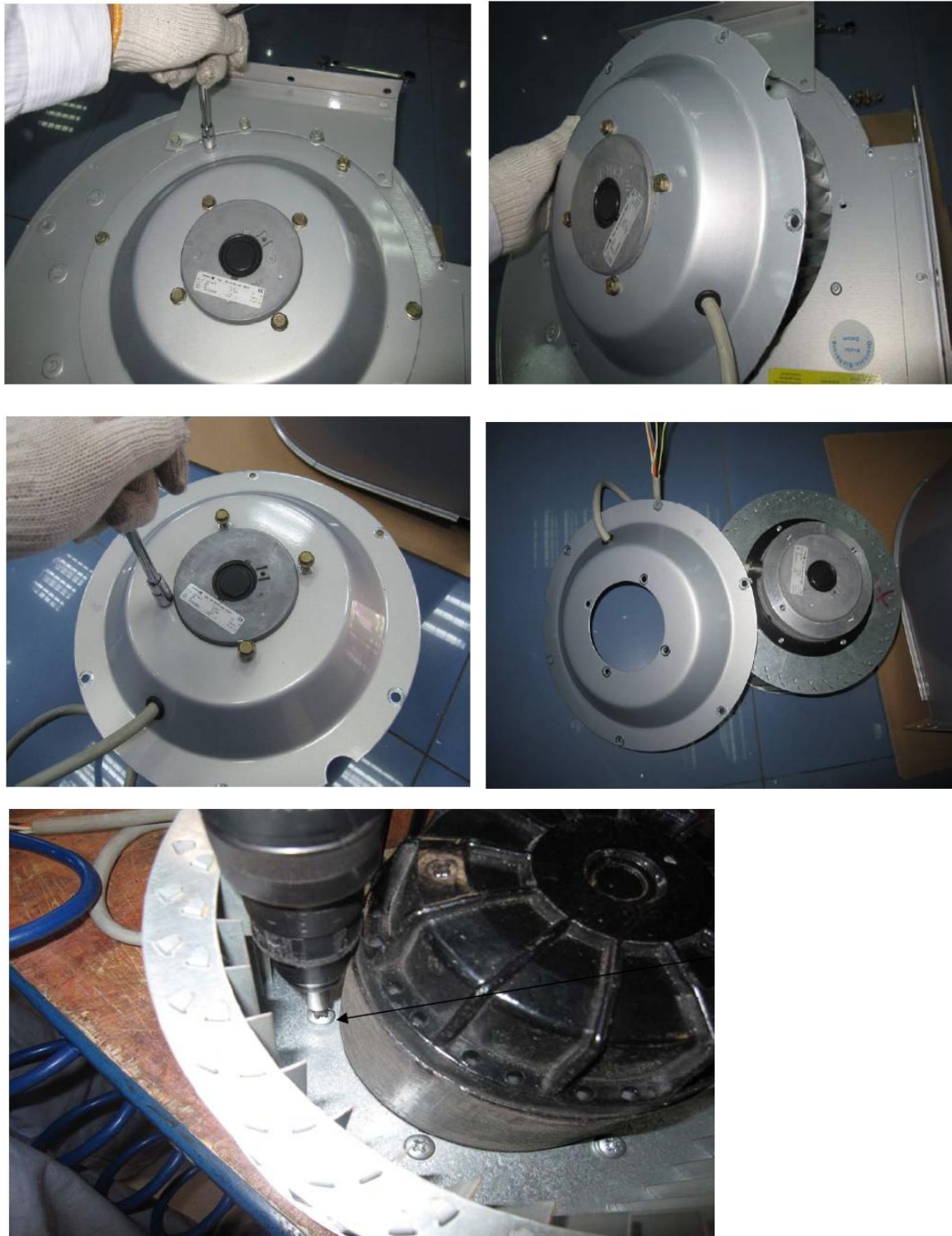
Figure 5.50-2 Replace supply air fan of saloon HVAC unit
