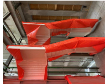
Inside building R13
