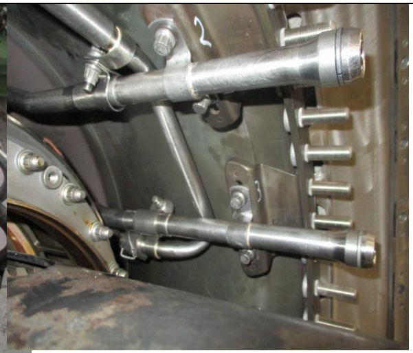
CRF oil manifold install per SB 308
