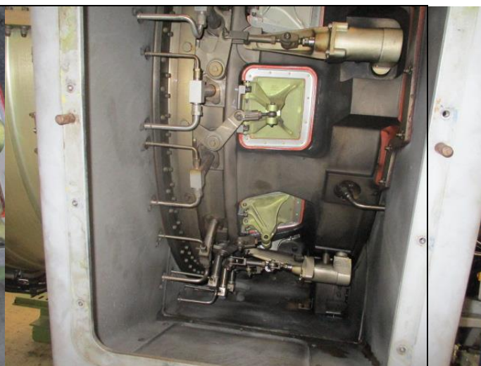
VBV doors replaced with new
