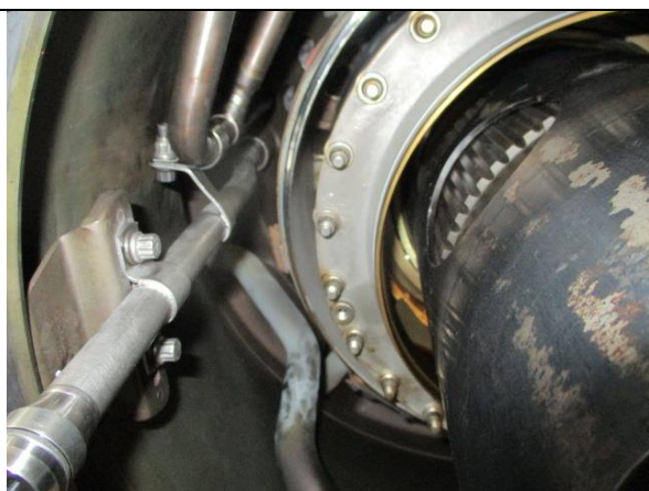
CRF oil manifold install per SB 308
