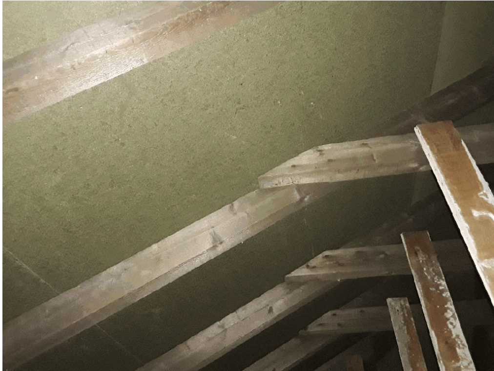
40B1 8E5, dakbeschothout
