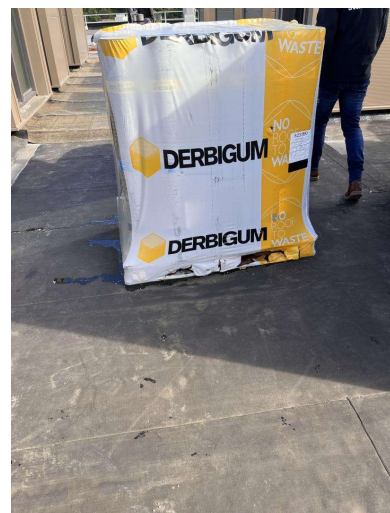
Afb. 9: pallet met rollen dakbedekking
