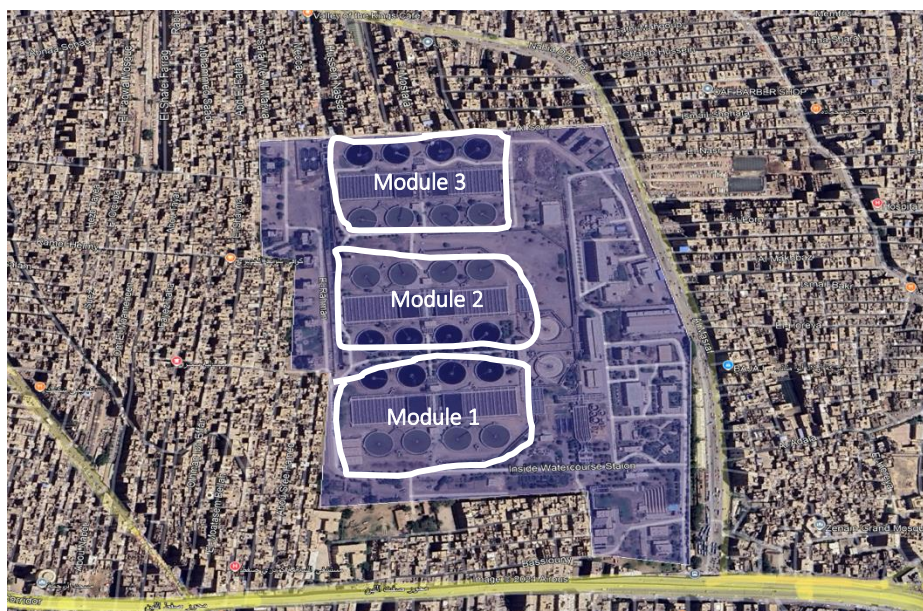
Figure 2. Aerial view of Zenien WWTP in GIZA governorate
