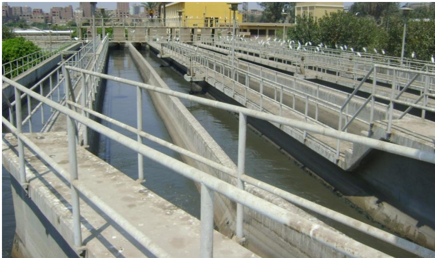
Grit Removal channels (No. 6 duty + 1 degritted)
