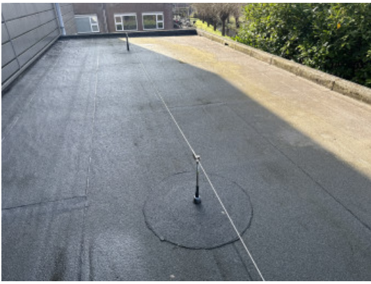
Lage dak links achter schoon
