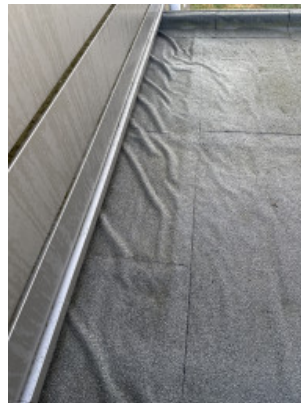
Lage dak links achter ploovorming
