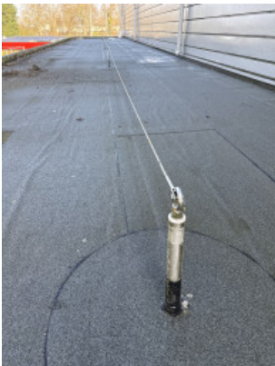
Lage dak links achter valbeveiliging
