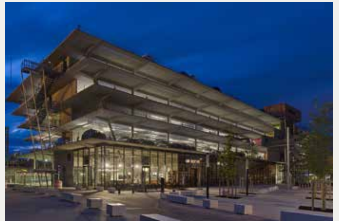
Lichte verdiepingen Parking P3 - Gare Saint Jean Belcier
