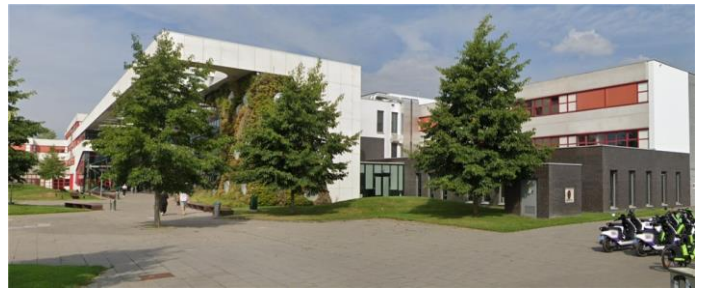
View East side on building F
