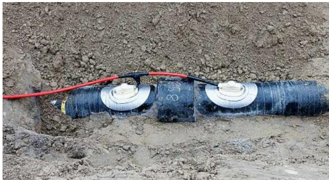
Figure 4: Installation of Ex-Spark Gap for Insulating Coupling
