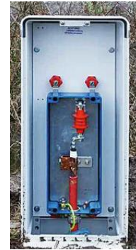
Figure 4: Installation of Ex-Spark Gap for Insulating Coupling
