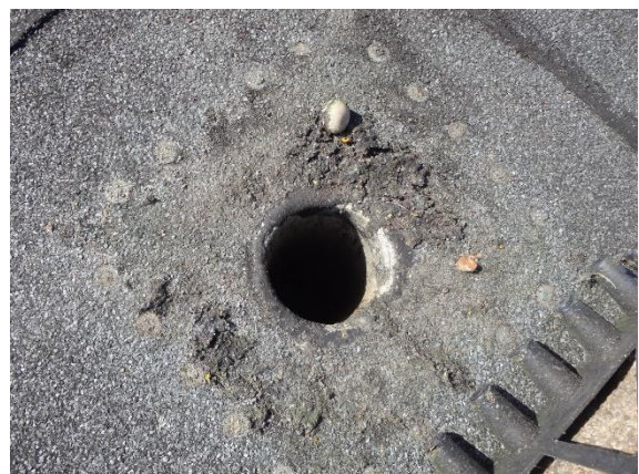
18: detail hemelwaterafvoer (onderuitloop)
