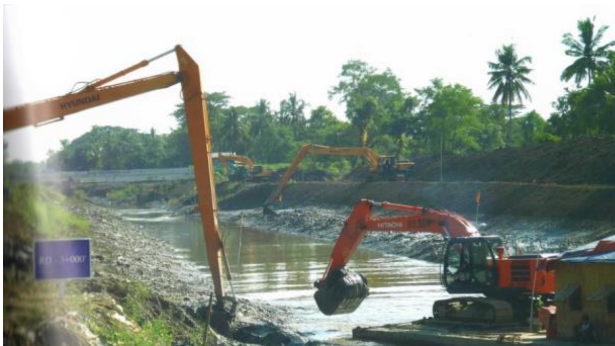
Figure 90: Picture of channel reconstruction works
