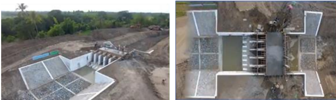
Figure 88: Example pictures of sluice structures
