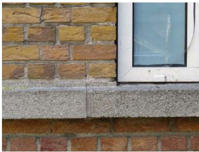
Incidentele haartrapscheuren in metselwerk =>
