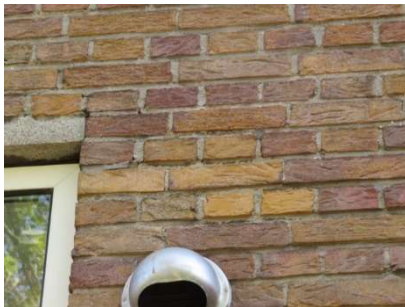
Incidentele haartrapscheuren in metselwerk =>
