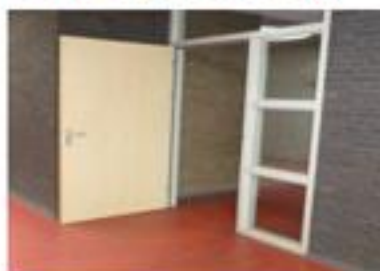
TOEGANG VANUIT SCHOOL
