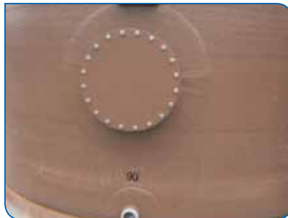
SERVICE LUIK IN WAND LAVAFILTER
