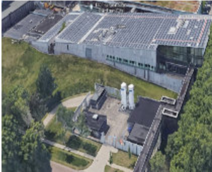
Flammable gas storage
