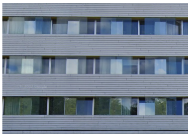
Studentenhuysvesting: glazen schuifpanelen, houten latten
