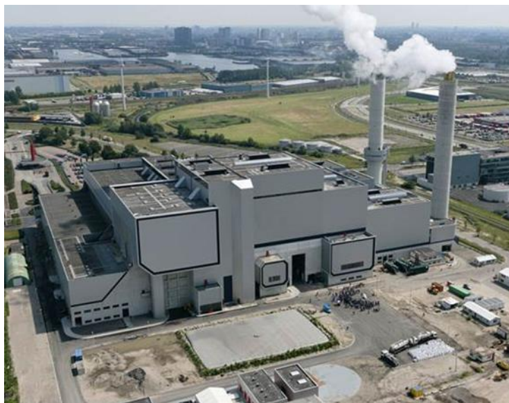
Figure 1-1 AEB waste incineration plant (source: internet/public domain)
