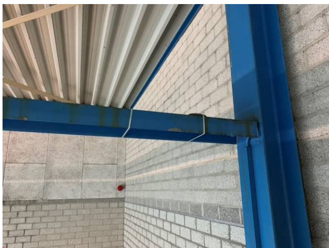
Corrosievorming vakwerkspanten in as 26 en as 27
