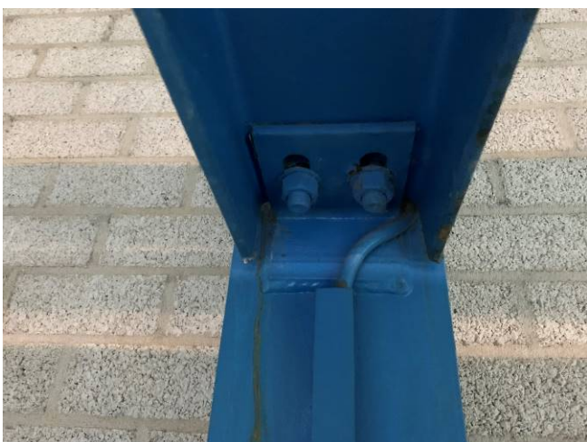
Corrosievorming vakwerkspanten in as 26 en as 27
