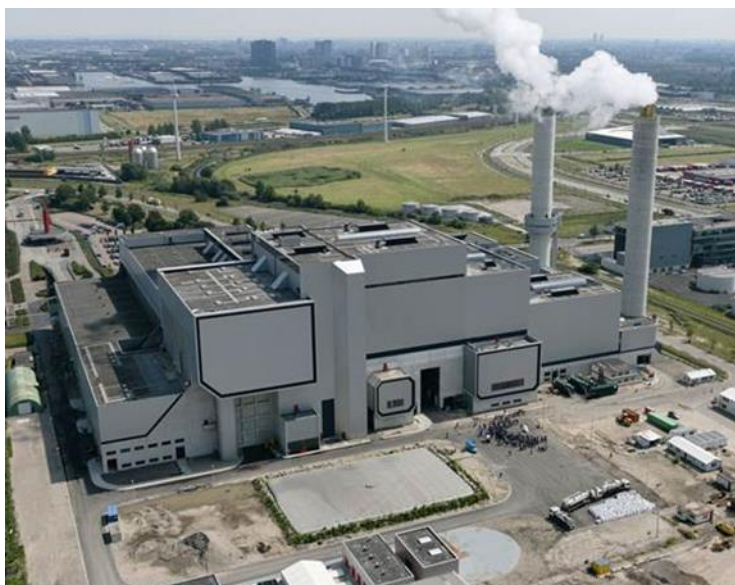
Figure 1-1 AEB waste incineration plant (source: internet/public domain)
