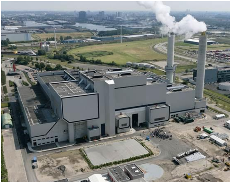
Figure 1-1 AEB waste incineration plant (source: internet/public domain)
