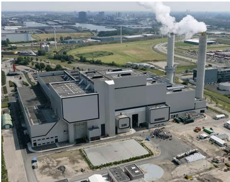
Figure 1-1 AEB waste incineration plant (source: internet/public domain)
