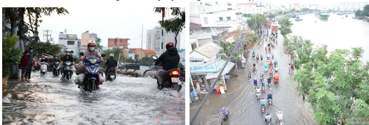
Figure 2. Tidal flooding in Hochiminh city, 2021
