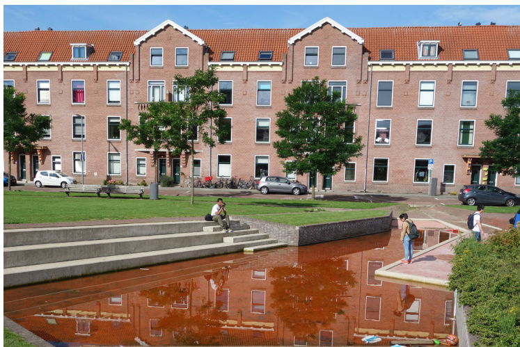
Rotterdam - Bellamyplein - waterberging
