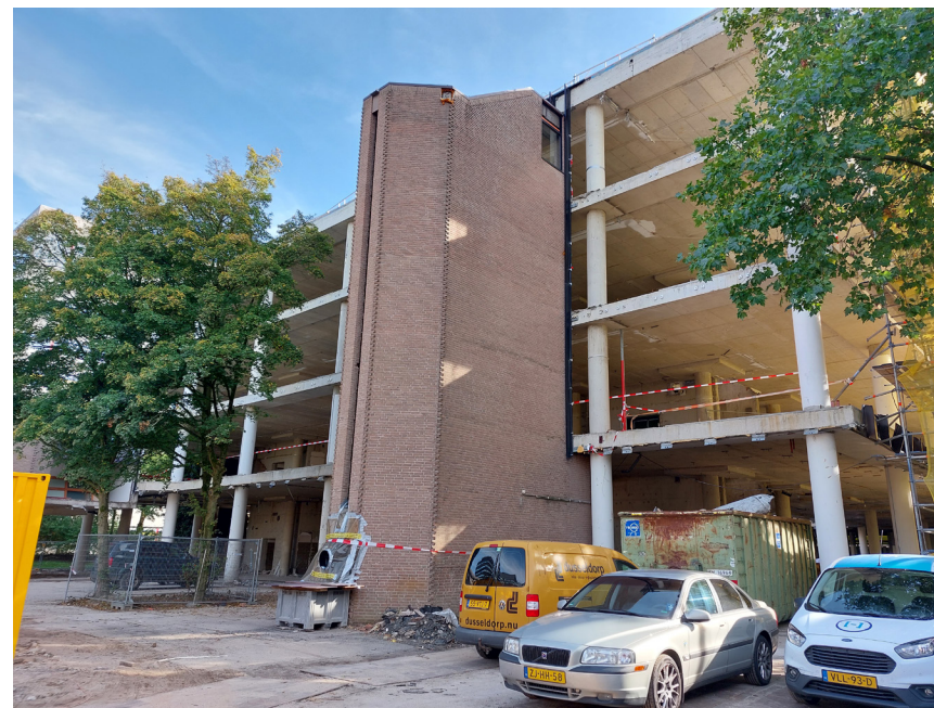
Te slopen extern trappenhuis
