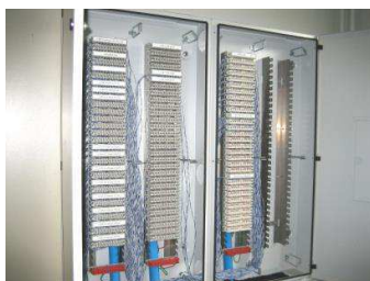
Figuur 5: LSA+ wandverdeler
