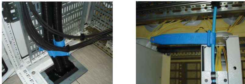
Figuur 4: Labeling multiduct NAFIN
