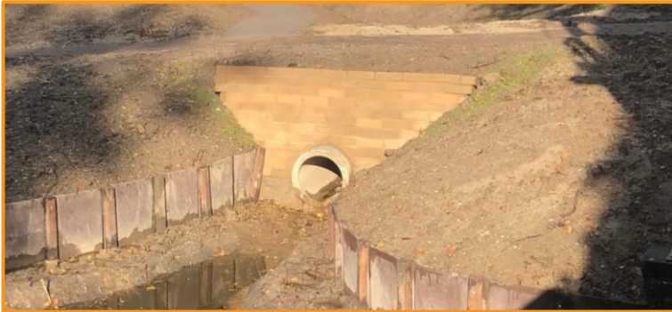
Figure 8 Revetment from compressed stabilised sediment under construction
