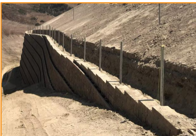
Figure 9 Reinforced soil retaining wall with brick facing (Belgard Commercial)
