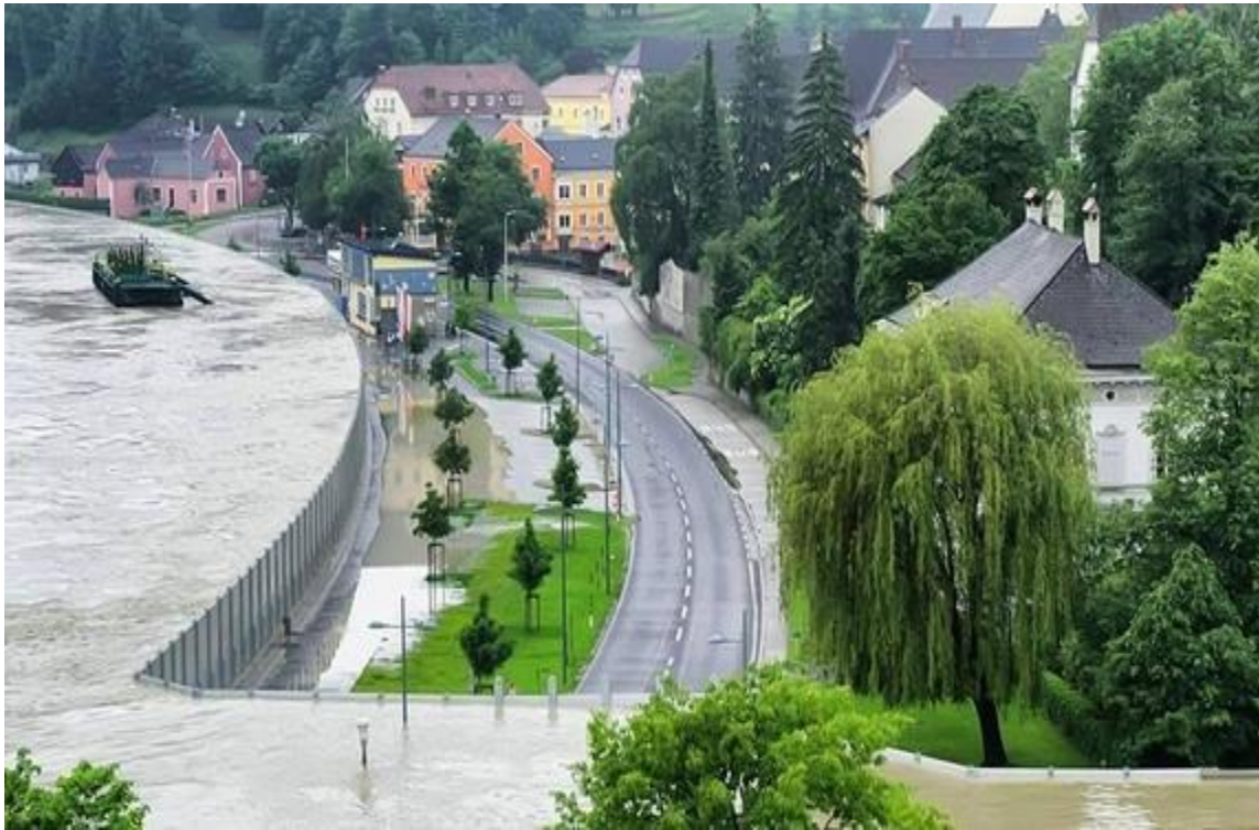
Figure 4.12 Residents may feel safe, but the potential impact of failing embankments is higher compared to unconfined rivers
