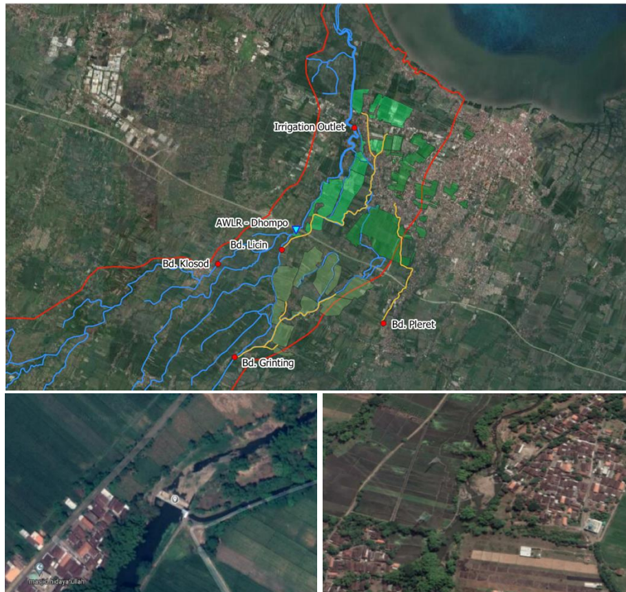
Figure 7-9 River diversion above AWLR Dhompo (Intake Grinting, bottom left and Intake Licin, bottom right) Source: Google Maps
