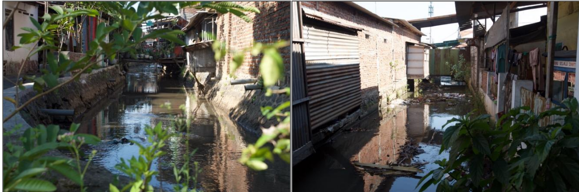
Figure 2.18. Domestic and industrial wastewater disposed directly into the Licin irrigation channels in Kraton (source: author)
