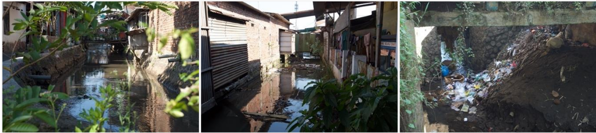
Figure 5.11. Irrigation channels are also used to discharge stormwater, although discharge capacities reduce due to combined decreased channel width/depth and accumulated solid waste trapped near outflows (gates)
