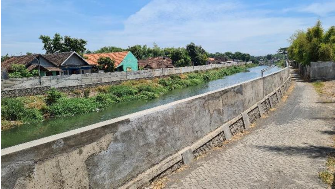
Figure 6 Newly constructed and raised (1.5 m) concrete river embankment near Kraton Bridge.
