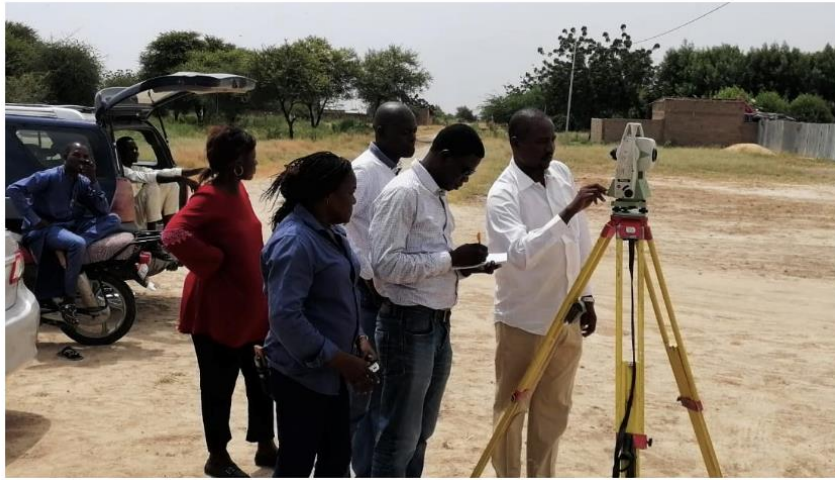
Figure 14: Demonstration 1 – Traditional Surveying in the field
