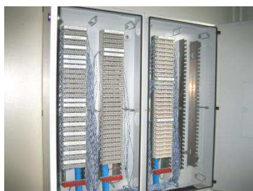
Figuur 5: LSA+ wandverdeler
