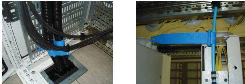
Figuur 4: Labeling multiduct NAFIN
