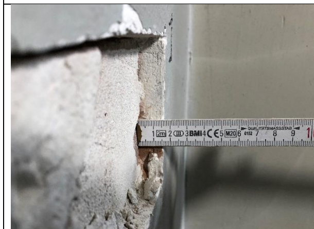
39. Laagdikte stucmortel is 16 mm.
