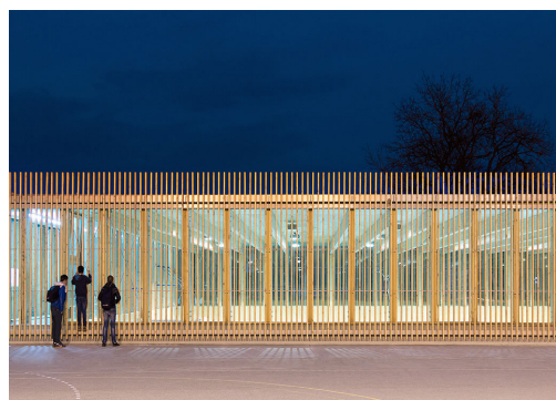
Transparante gevel Elementary school sports hall, Obrenovac Jovan Mitrović
