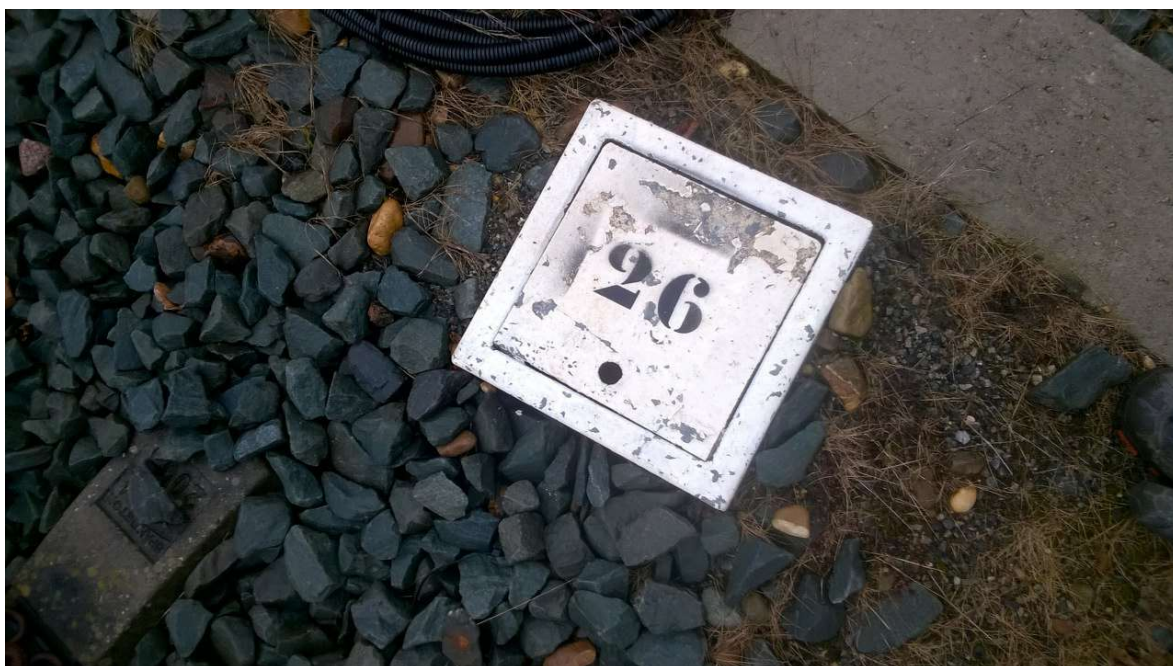
Figuur 22 Hydrant/Was & vulhydrant
