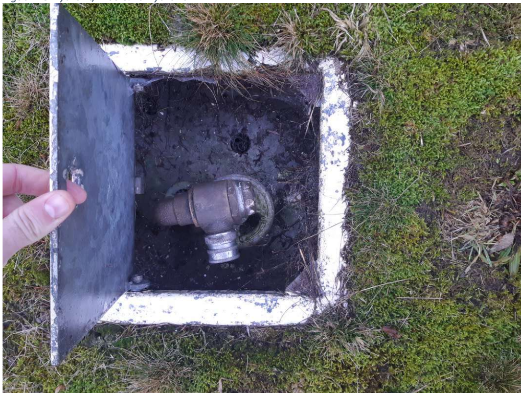
Figuur 26 Hydrant, Was & vulhydrant type NS
