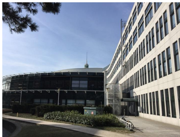
Left building C, right south façade of building B
