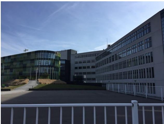
Northern facades of buildings Db, Da and A
