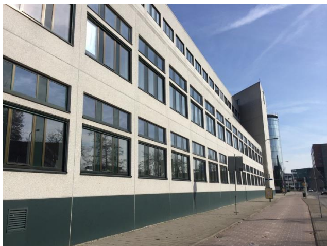
South façade of building A
