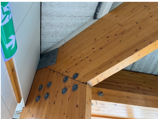
Foto 4: Detail hoekverbinding houten spant.
