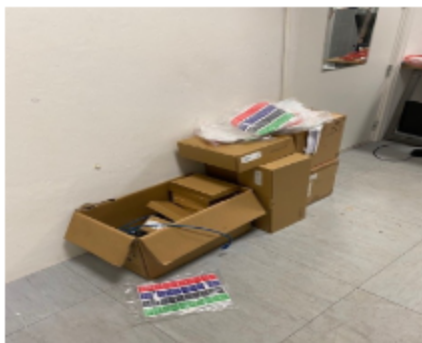
Server room storage
