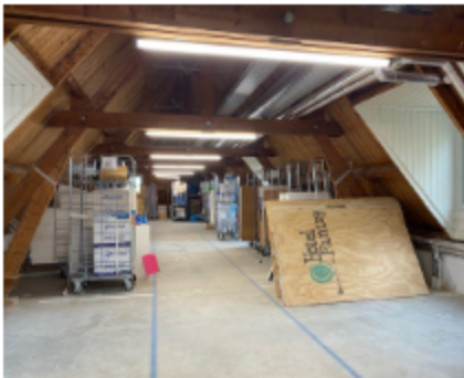
Wooden attic of monastery building
