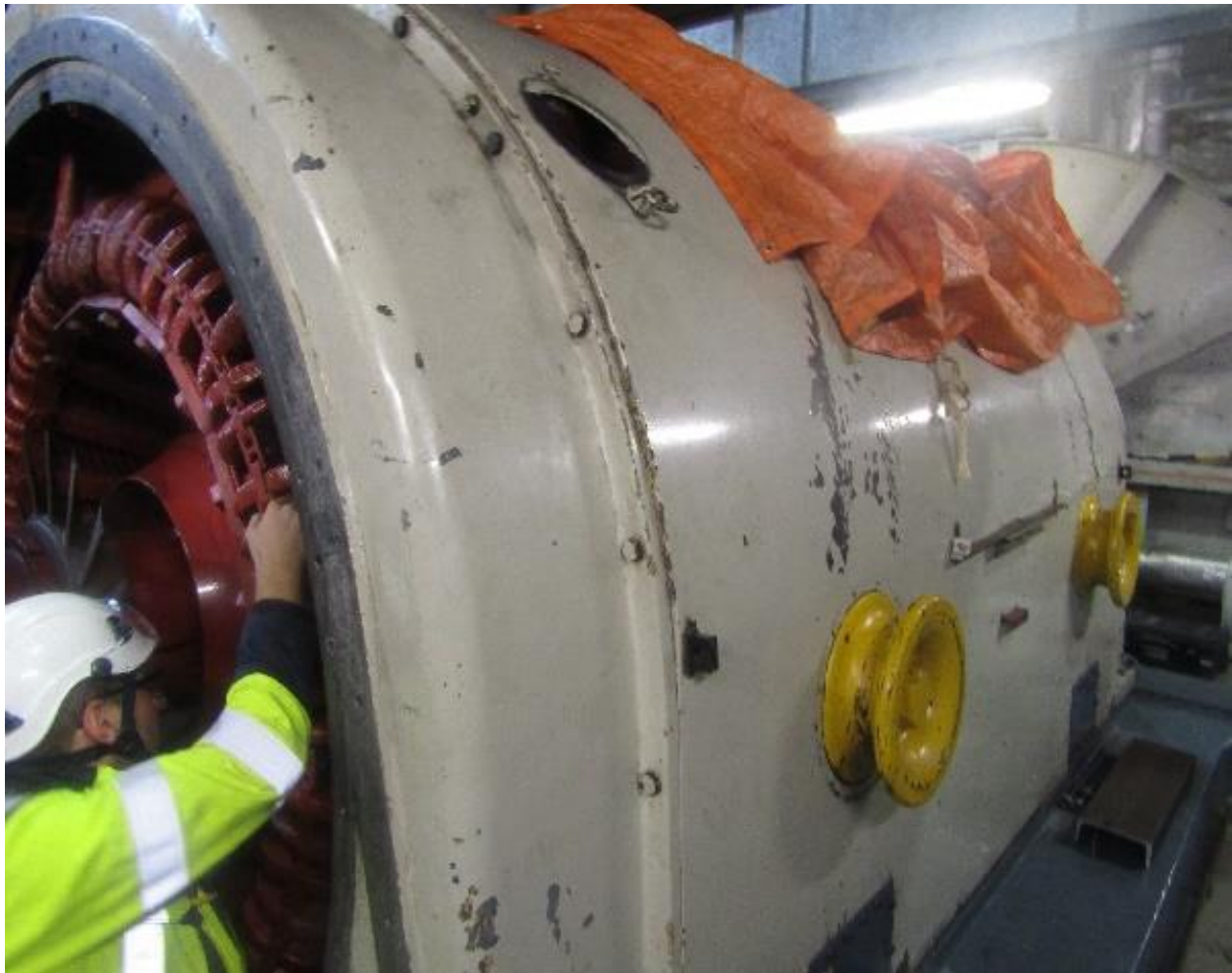
Statorhousing with liftingpoints
