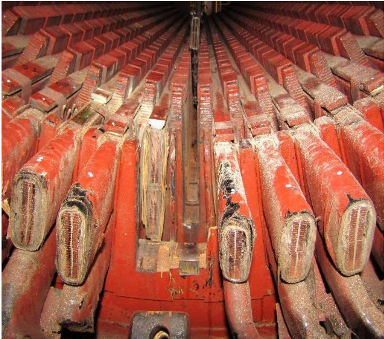
Top – and bottom bar partly removed for investigation
