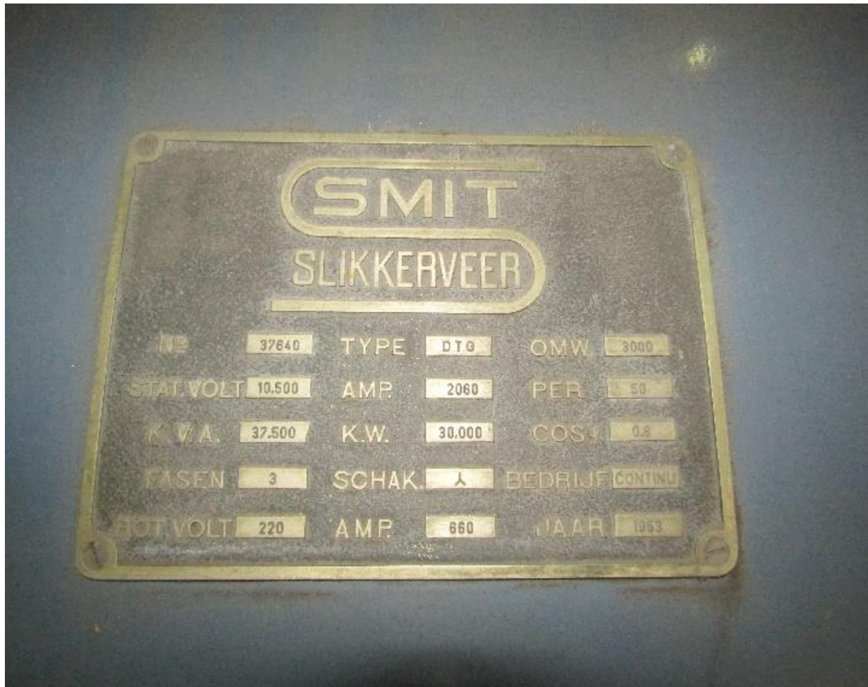
Tag plate spare stator at The Hague
