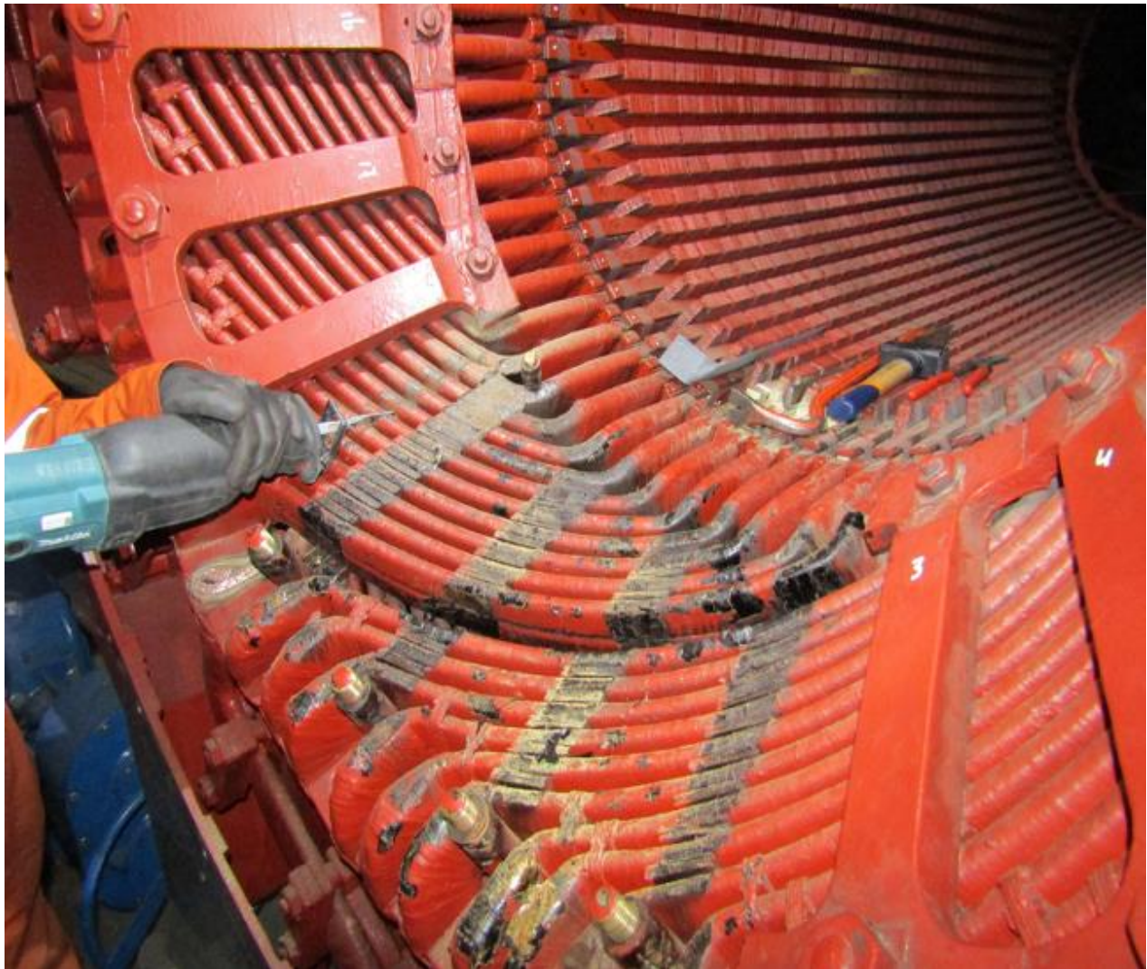
Windinghead CE during dismantling of the stator bars
